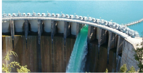
Kerr Dam in Montana
